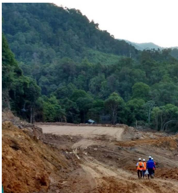
Sealed Stockpile Pad Completed
