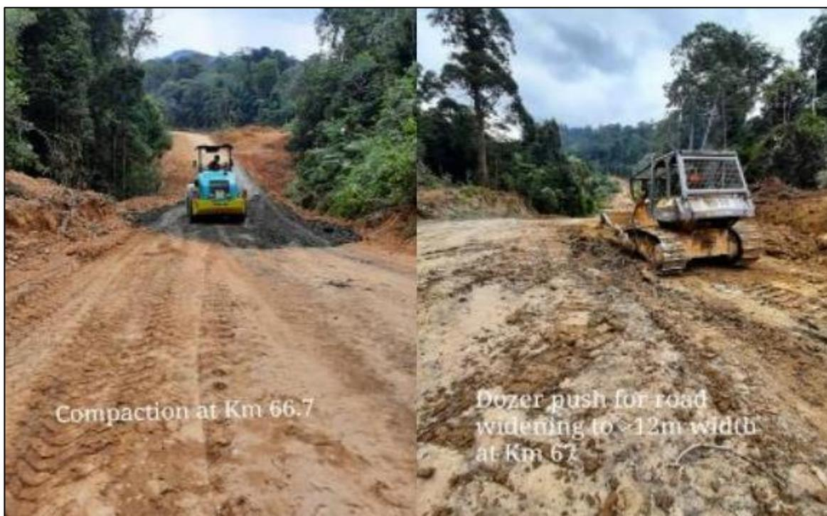
Figure 1 – BBM Road Construction (source: CKA ASX announcement 9<sup>th</sup> August 2021)
